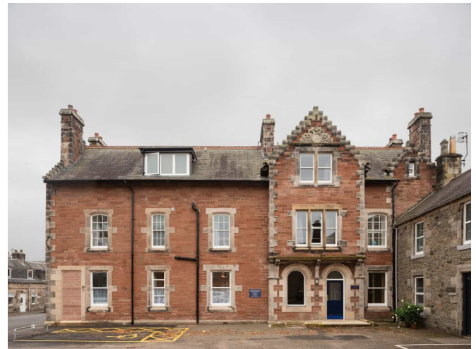
Images: The Old Police Station. John Gilbert Architects / SOSCH - ©Tom Manley
