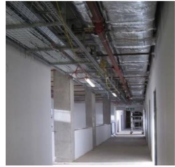
Images (L) The FF&E3D model was utilised for stakeholder consultation, RDD sign off, and coordination with the design models. (above) Coordinated MEP systems and framing were modelled digitally and fabricated off site. Model data was used to check tolerances and simulate virtual installation sequences.
